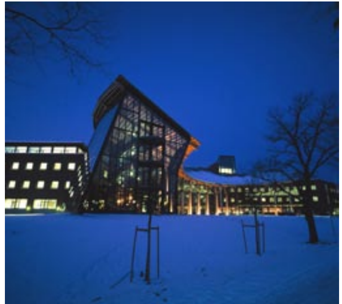
Statoil office in Trondheim, Norway
